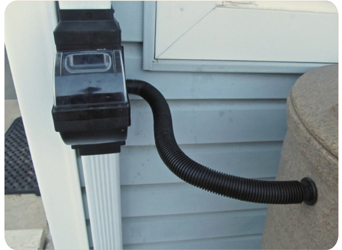
Diverters allow for easy maintenance of your rain barrel
