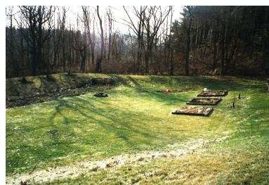
Figure 4. Berms direct the surface runoff flow into a large, flat area, where water can infiltrate into the ground. The presence of surface vegetation helps to slow the surface runoff and reduce erosion.
