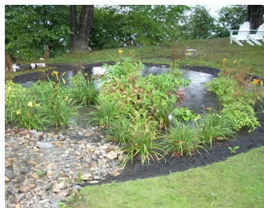
Figure 1. Rainscaping at work, transferring runoff from the rocky higher ground, where friction slows it down. The runoff spreads out over the lower ground and soaks into the permeable ground surface.
