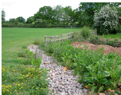
Figure 3. (left) French Drain Under Construction and (right) Established
