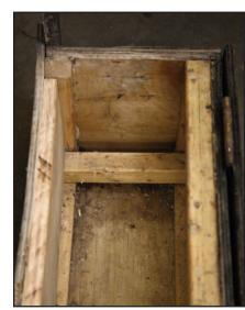
You should brace the box as in the picture since unsupported plywood warps. You need something to hold the paper off the bottom of the box and keep it dry; the bracing does that too. The roll of paper lies on the cross-braces and unrolls at the front so it has straight-up path to the crossbar.
