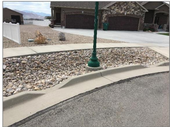
Figure 8: Curb cuts to a rock lined swale.
