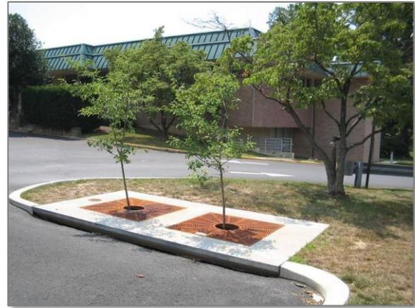
**Figure 13: Proprietary tree box filter**
