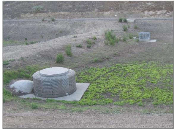
Figure 4: Multi-stage overflow outlet with trash screen
