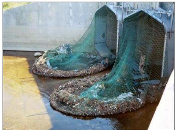
Figure 5: End-of-pipe trash netting
