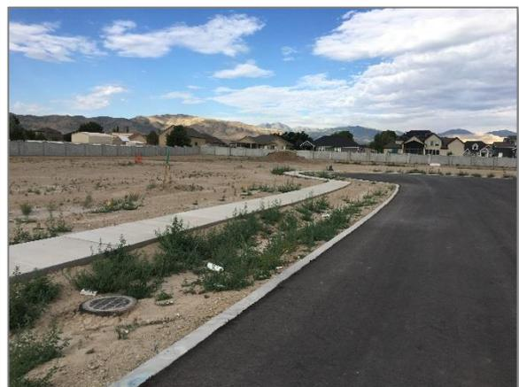
Figure 12: A vegetated swale that will provide pretreatment for a dry well.
