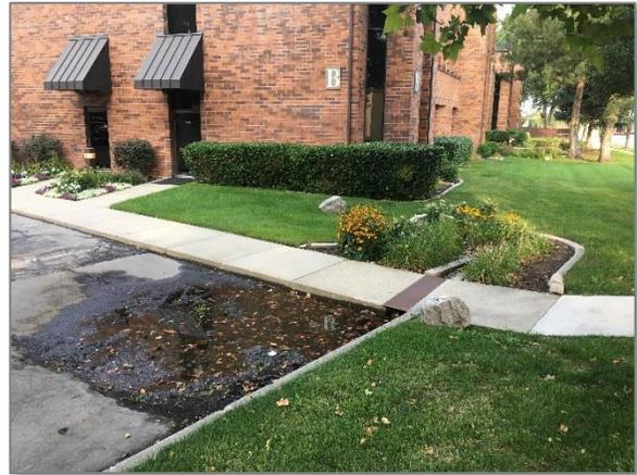
Figure 11: Standing water after a rain event at a bioretention BMP.
