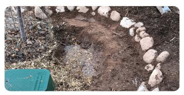
Installing earthworks for a gravity-fed graywater system in Moab, UT (pipe outlet into green mulch shield). Credit - Roslynn Brain McCann
