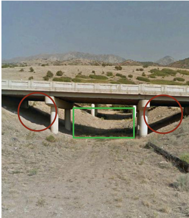
Figure 2.118 Wildlife underpass recommendations. Green box showing the area complying with recommendations. Red circles showing areas that need improvement.
