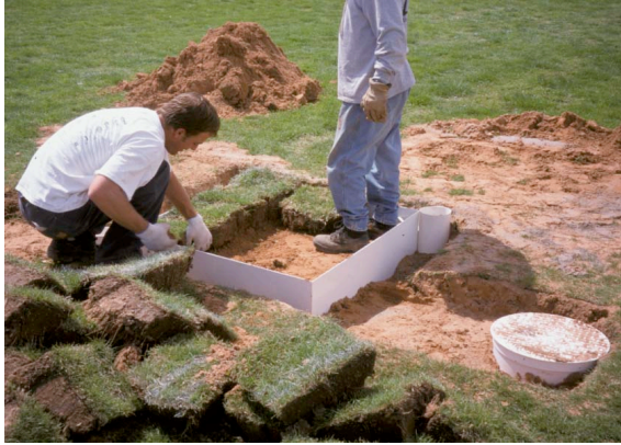
FIGURE 4. PLACEMENT OF SOD IN PARTIALLY INSTALLED LYSIMETER (SOUTHGATE, APR 2004)
