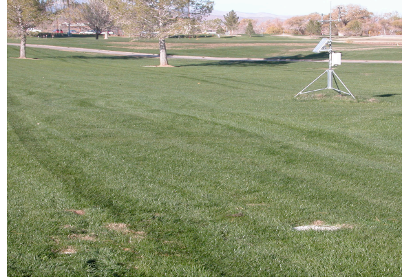
FIGURE 5. FINISHED LYSIMETER INSTALLATION (SOUTHGATE, DEC. 2004)
