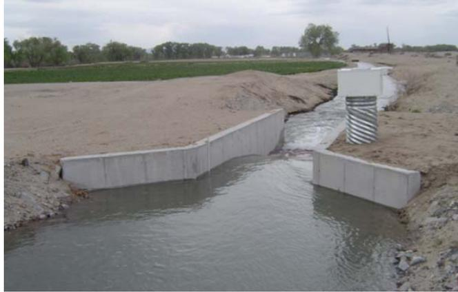
Figure 6. Standard TCID Replogle flume with water flowing
