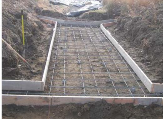
Figure 3. Framework and steel for the foundation
