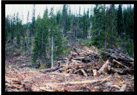
Keep slash pile free from dirt and other debris. This pile will burn cleanly and leave little residue.
