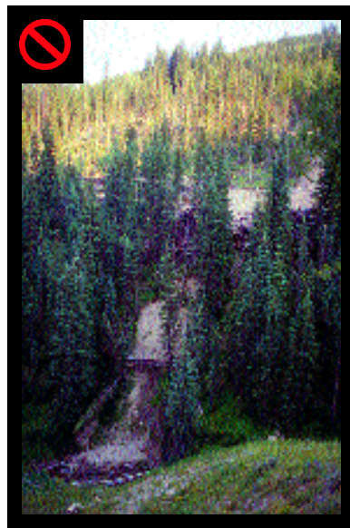
Avoid perched landings which may fail and cause substantial erosion problems.
