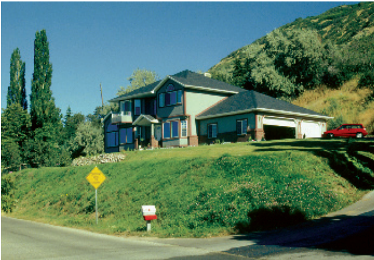
This home has good, wide firewise landscaping within much of its home ignition zone. Its Zone 1 is “clean and green”.
