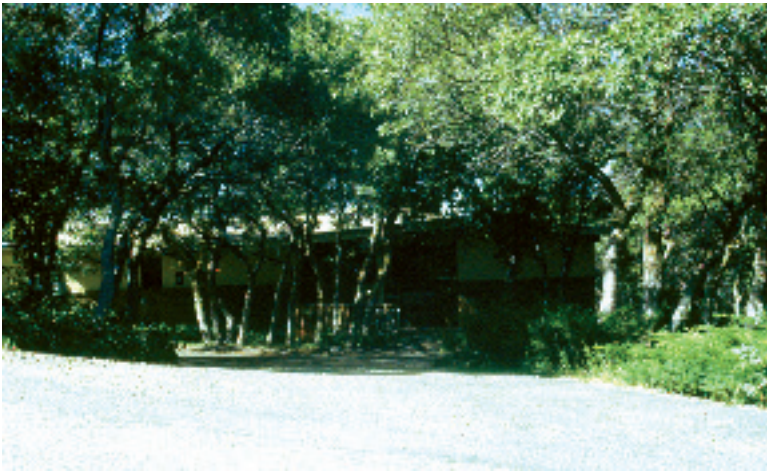
Although this home close to the road, its Zone 1 landscaping is not firewise, with highly flammable oak trees overhanging the roof.
