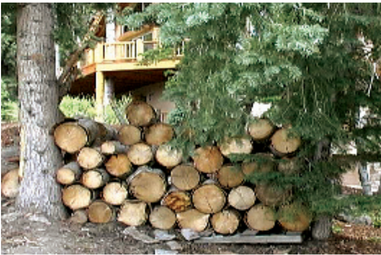
This woodpile should be moved at least 100 feet away from the house. Notice the unenclosed deck and tree growing up through the deck – both increase risk from a wildfire.
