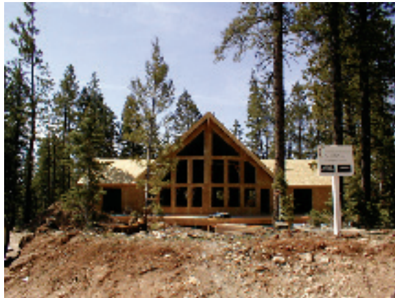
New construction in the wildland-urban interface.
