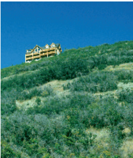
Placement of this house on top of a Gambel oak-covered ridge puts it at greater risk from wildfire, along with its wood decks.
