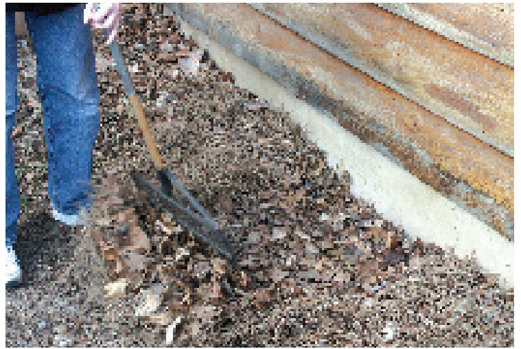
Rake and remove dead leaves, needles and other debris from wood structures.
