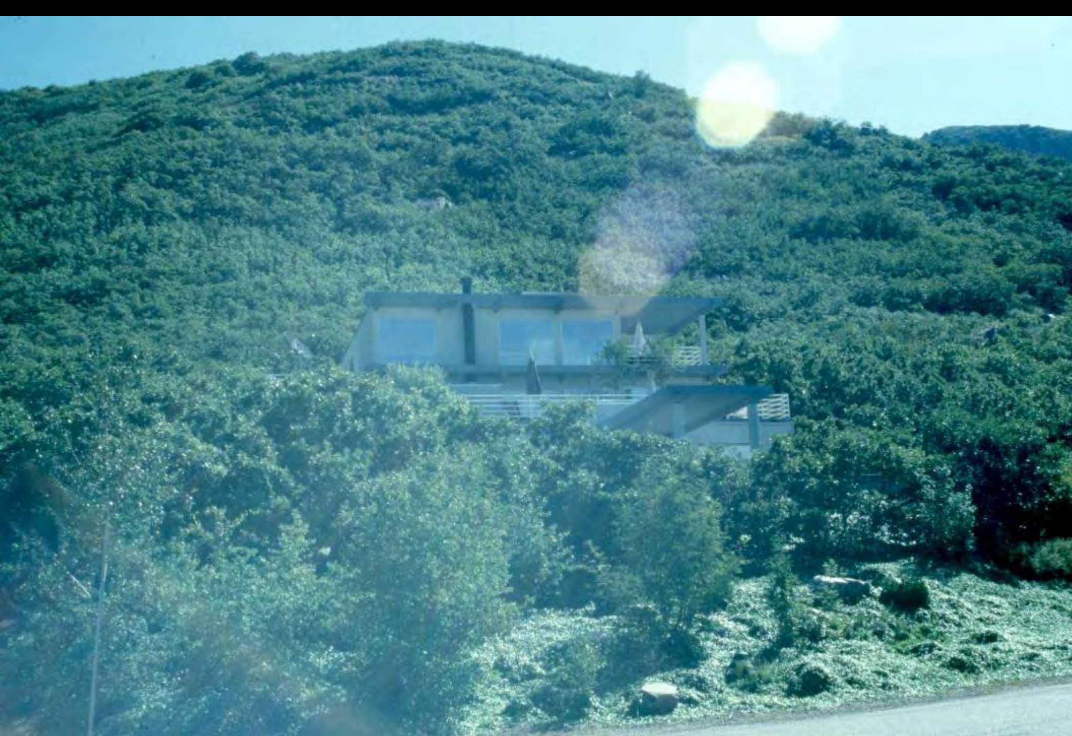
House in oak (Uintah, UT)
