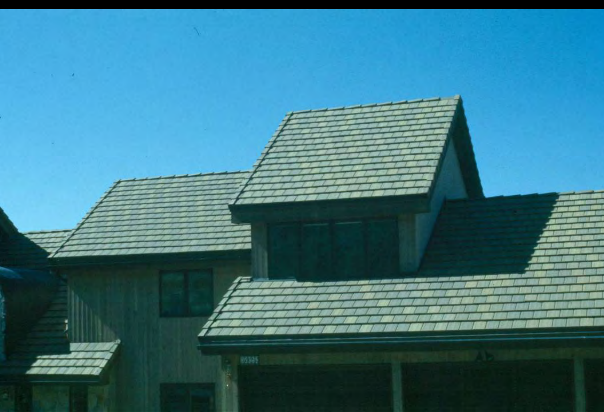
Class A roof, boxed eaves (Uintah, UT)
