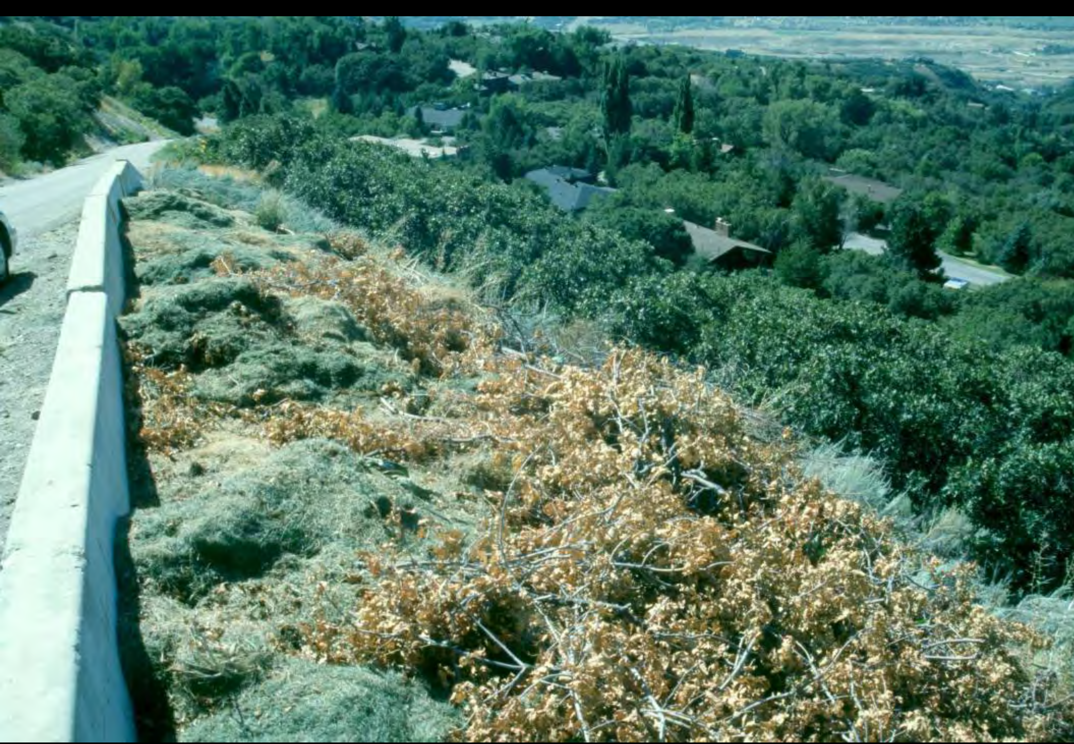
Debris along road (Uintah, UT)
