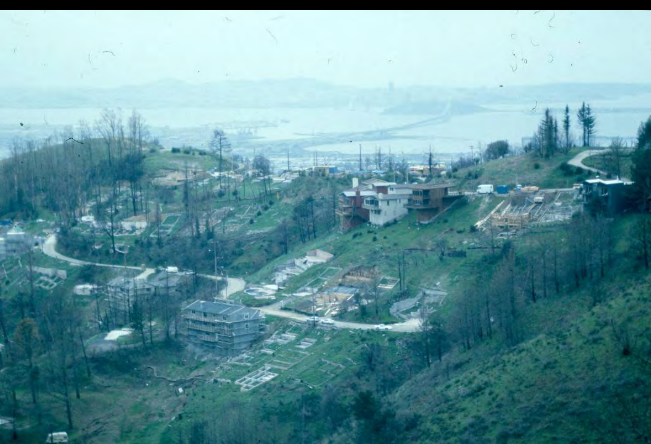
Berkeley Hills rebuilding, 2/93
