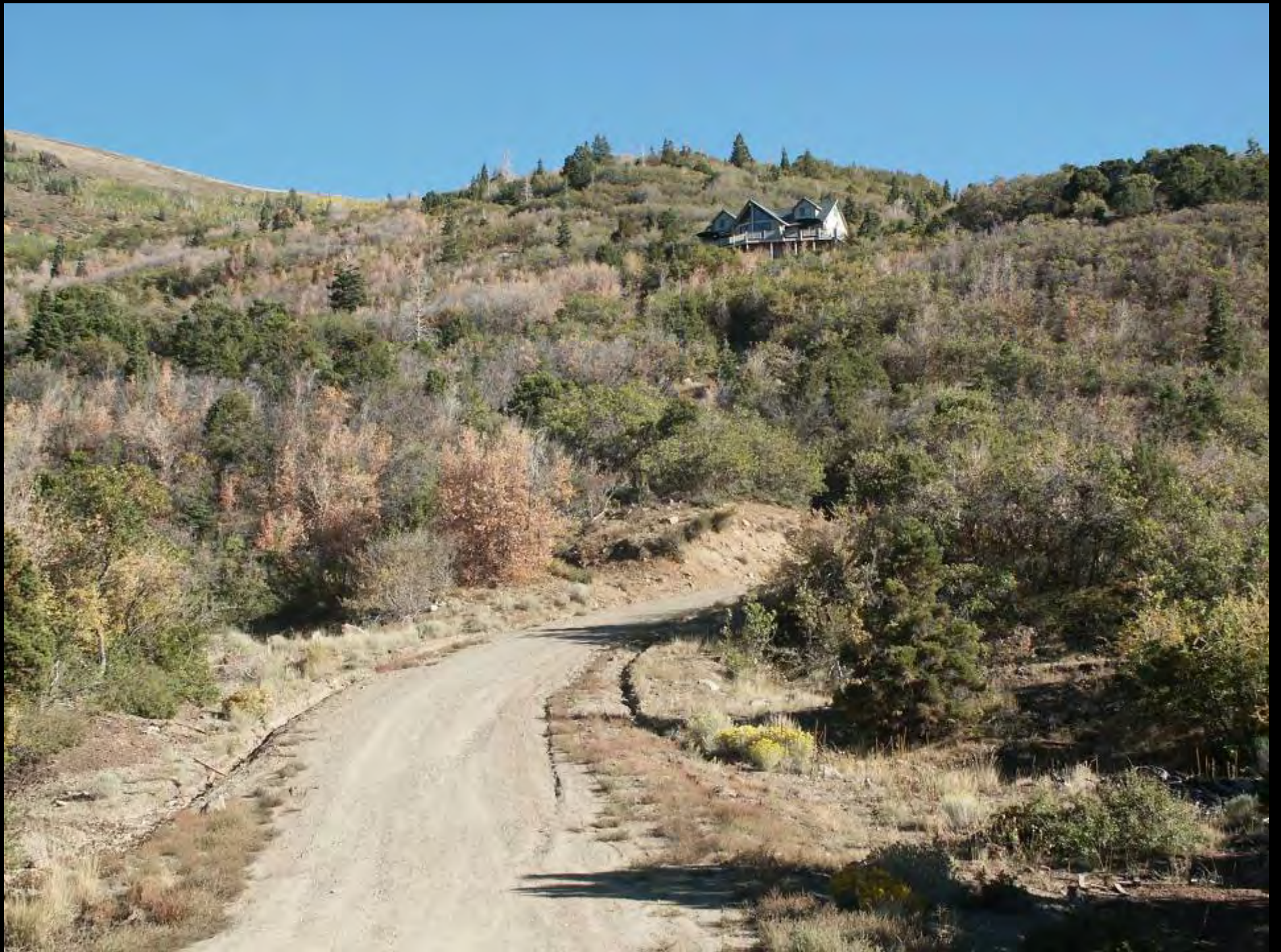
Steep, poor road (Cedar Highlands, UT)
