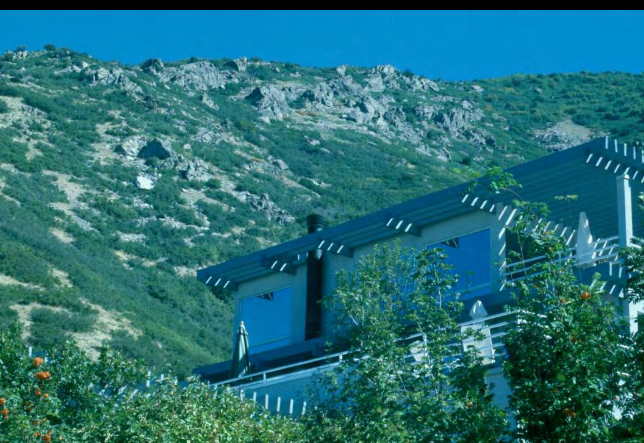
Screened chimney (Uintah, UT)
