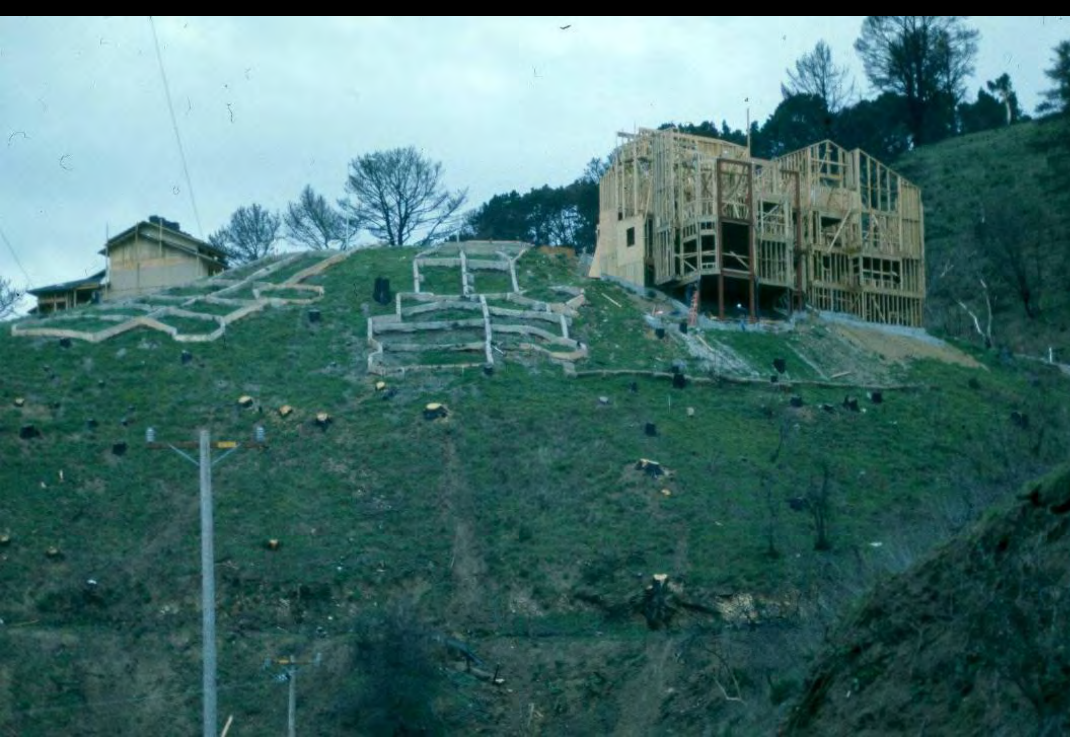
Berkeley Hills rebuilding, 2/93
