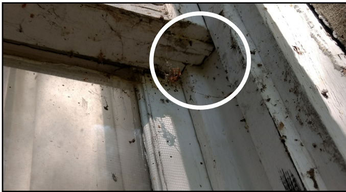
Fig 7. Elm seed bugs easily enter structures through gaps in the window frames.
