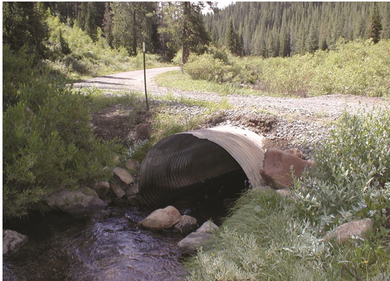
A properly sized and placed culvert will handle 50 year flood events and allow safe fish passage.
