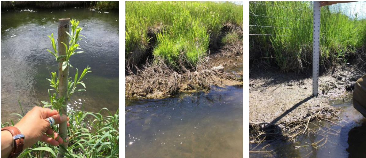
From left to right: a surviving planted willow, an installed streambank revetment, and sediment accumulating behind a revetment.
