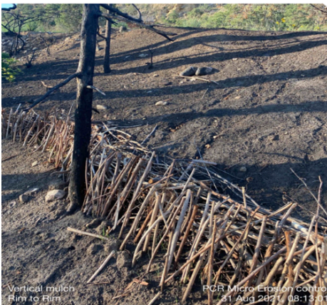
Figure 4. Terracing With On-Site Material to Control Soil Erosion
