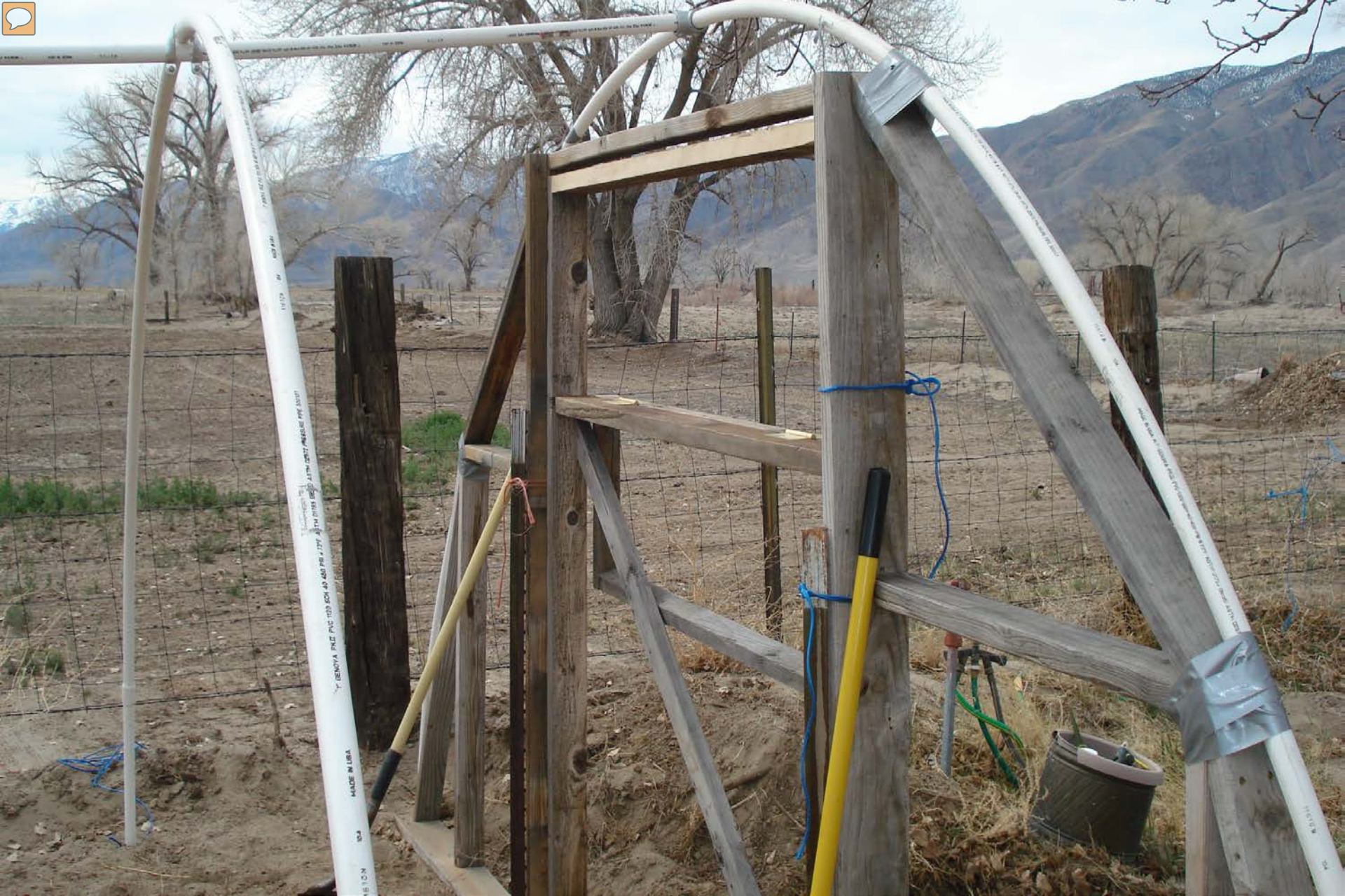
Vented hoop house door – “T” post attachments
