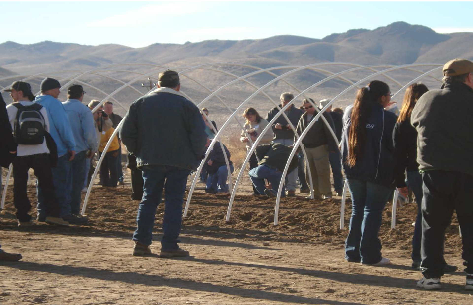
Installing PVC hoops
