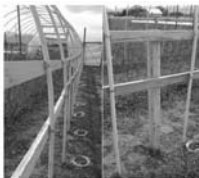
Figure 2. 2x4 side supports connected to PVC straps and 4x4 anchors. Cables will be attached over the tunnel to further secure the plants.
