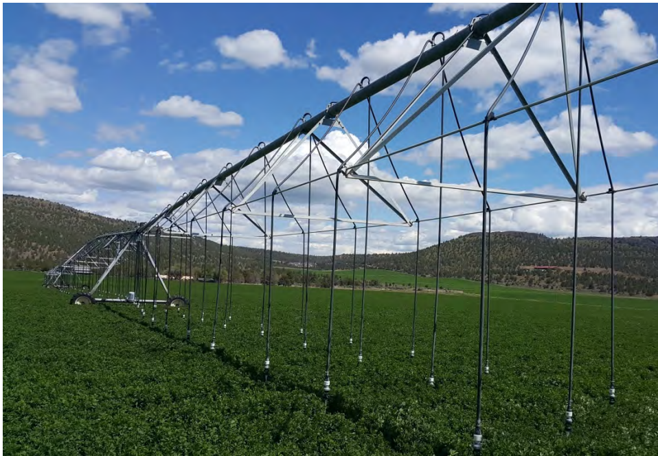
Figure 52. LESA on a center pivot that uses three drops per pivot outlet.
