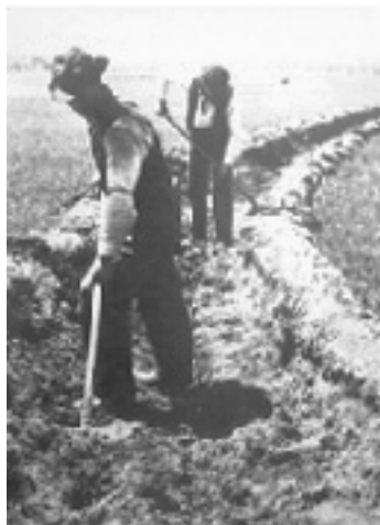
Figure 4. Pioneers Digging Irrigation Ditch. (Hooton, 1999)
