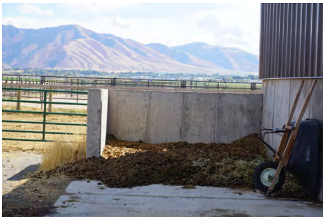
Figure 2. Manure storage area with a concrete pad and sidewalls
