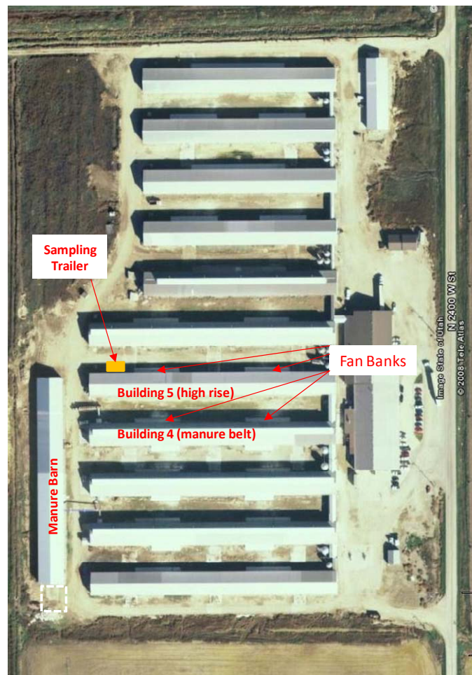
Figure 1. Poultry facility site layout (annotated GoogleEarth™, 2010).
