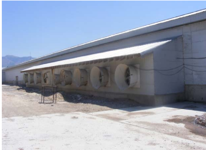
Figure 2. High-rise building (Building 5) external exhaust fans.
