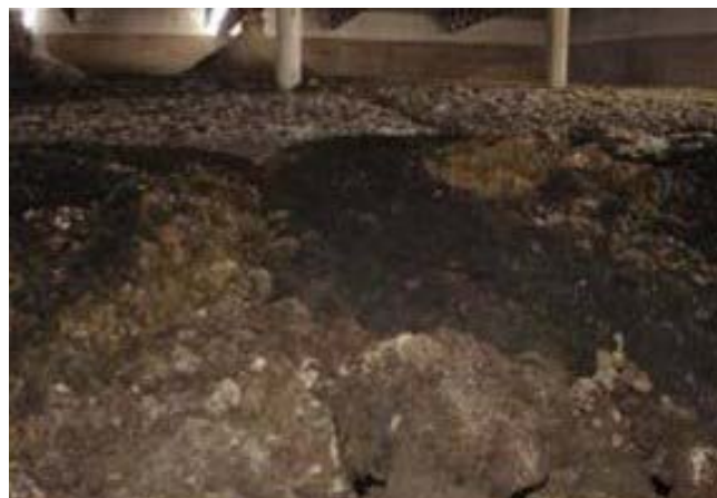
Figure 7. Internal view of manure storage barn (manure-belt depository).
