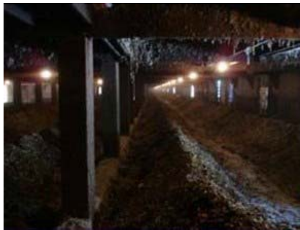
Figure 5. Internal view of manure storage in the high-rise building (Building 5).
