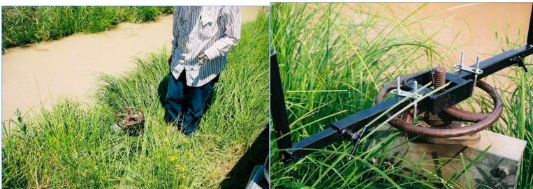
Figure 1. Handles added to irrigation headgate to
