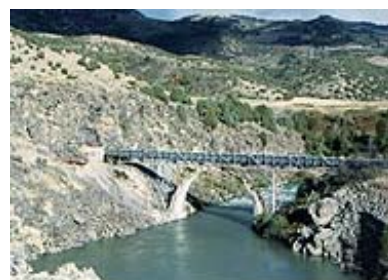
Last Chance Canal, Gorge and Bridge (Photo © 1999 A. Crane)
