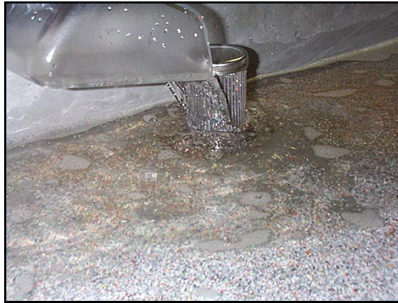
Outlet filter keeps grit out of water tank below. Clear filter by rotating swirling, or washing it with water.
