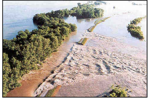
Levees can fail or make floods worse downstream. Picture from flip chart shows failure of levees.
