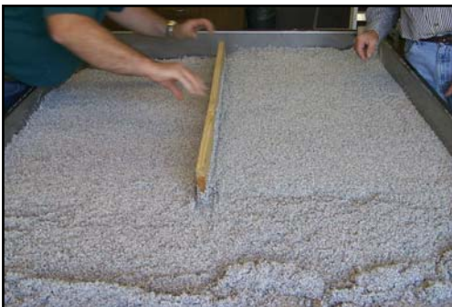
Screed board is used to smooth and level grit.
