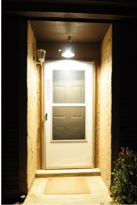
Figure 20-A 5W LED bulb in a fully shielded fixture. (NPS/Zach Schierl)
