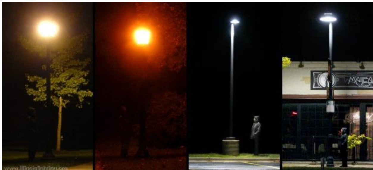
Figure 21-Photographs of four streetlights at night, two unshielded (left), and two fully shielded (right). There is a person standing beneath each light, but the combination of glare and dark shadows created by the unshielded streetlights renders them nearly invisible. (Illinois Coalition for Responsible Outdoor Lighting)
