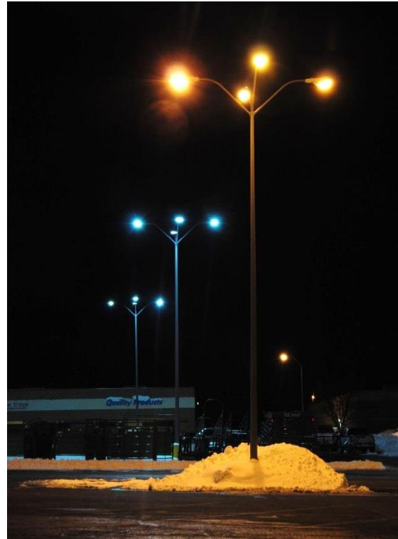
Figure 12-Parking lot lit by a combination of warm high-pressure sodium lamps (foreground) and cool LED lamps (background). (NPS/Zach Schierl)
