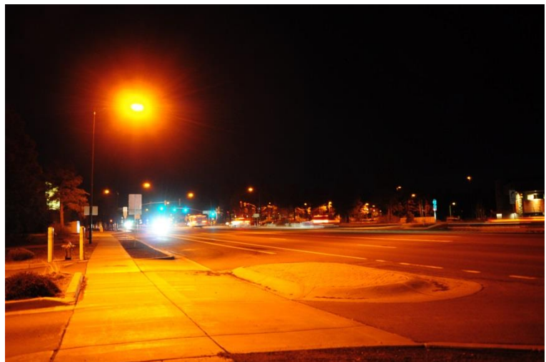
Figure 15-An arterial street in Flagstaff, AZ illuminated by narrow-band amber LED (NBA LED) streetlights. (Zach Schierl)
