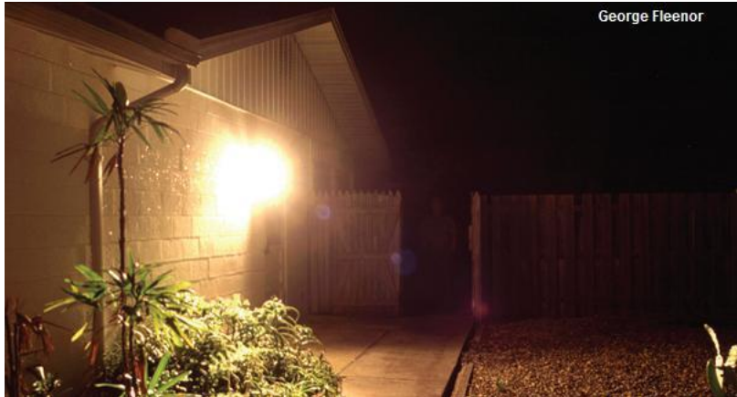
Figure 5-This unshielded floodlight on a residence is a classic example of glare. Note the human figure standing in the open gate. Glare prevents the eye from seeing into darker areas of the scene. (George Fleenor)
