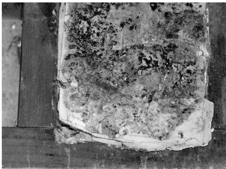
Figure 20-2. Mold hidden inside a wall
