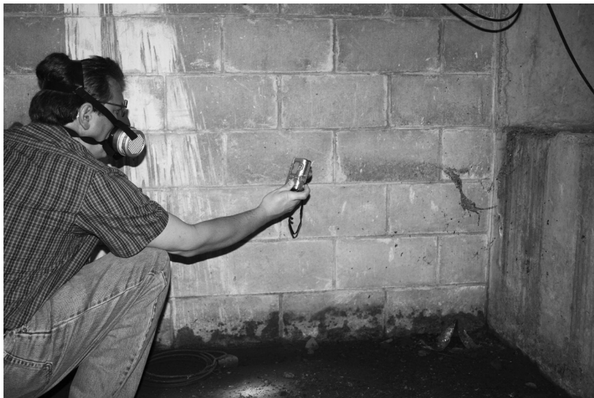
Figure 2-1. Inspect basements for signs of cracks or moisture.
