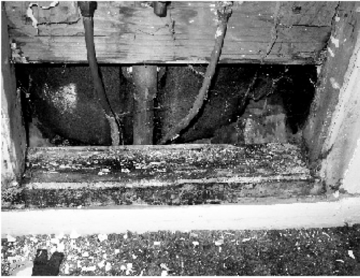
Figure 20-4. Wood damaged by moisture and mold.
