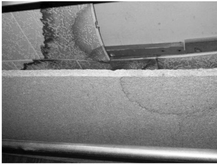
Figure 20-3. Ceiling tile damaged by moisture.
