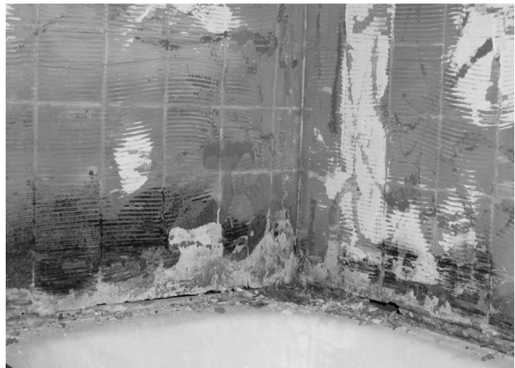
Figure 20-1. Mold on wall behind removed ceramic tiles
