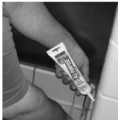
Figure 4-1. Applying caulk to cracks and crevices is one treatment strategy that will help reduce pest harborage and entry points.
