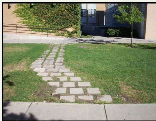
A brick path installed to hide a recurring compaction trail.
