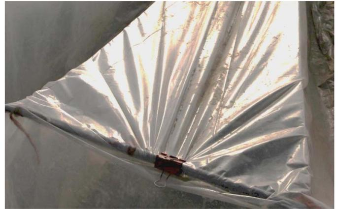
**Image 7.** Binder clip securing plastic to conduit frame.
