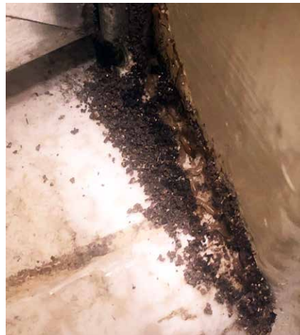
Left: Subterranean termites surrounded by clumpy debris, a common sign of termite infestations.
