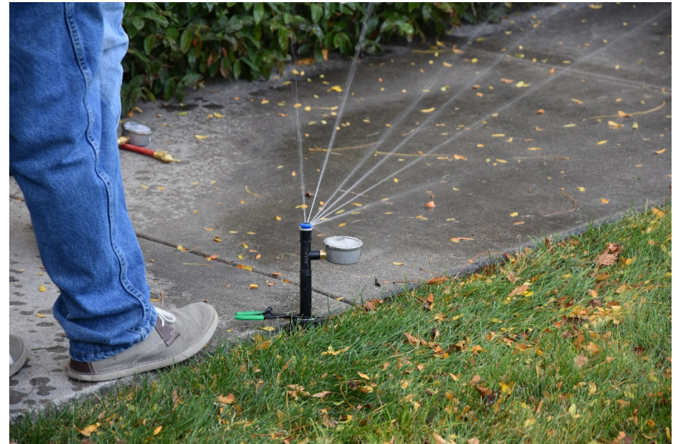
Testing water pressure on a sprinkler system (photo taken pre-COVID-19).
